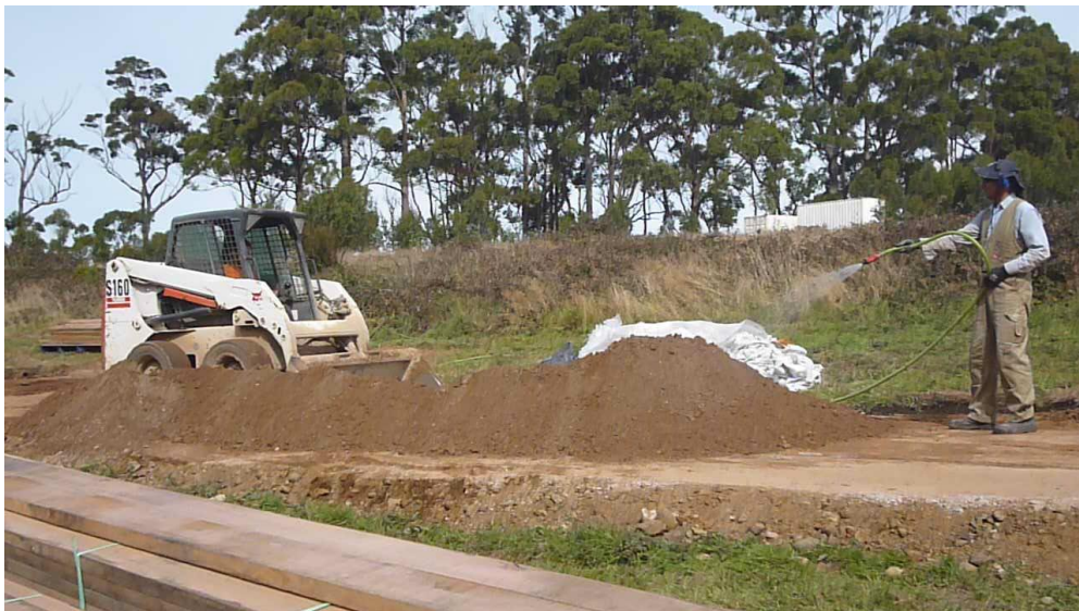
Mixing the material for the rammed earth walls
