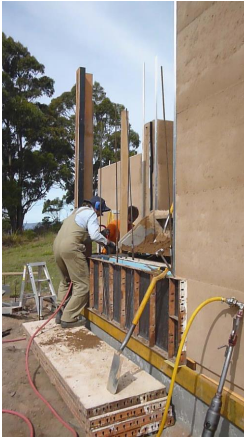
Mixing the material for the rammed earth walls
