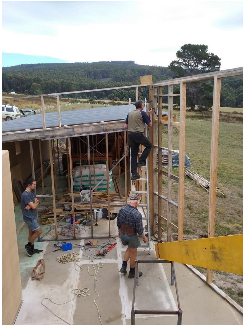
Stud frame installation and LVL main beam being installed:
