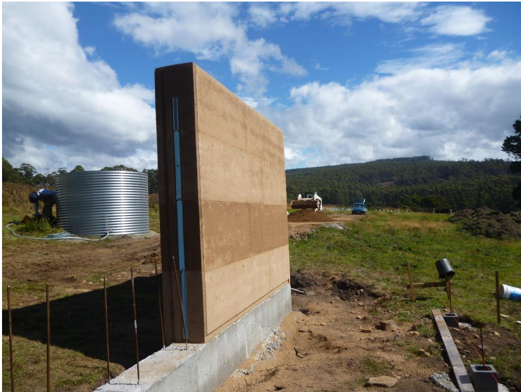
First section of the rammed earth wall going up. You can see the insulation inside the wall:
