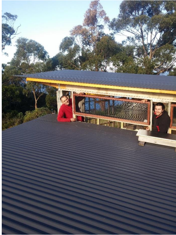
Bracing ply installed. Roof wrapped with foil adhered blanket insulation.
