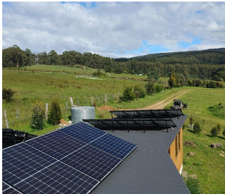
Solar panels are up
