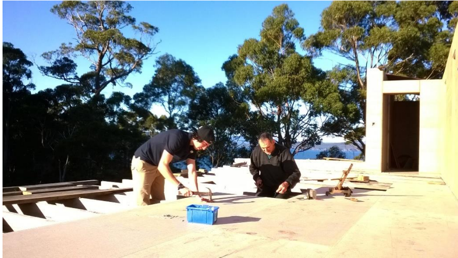
Yellow tongue sheet flooring being installed
